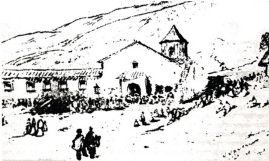
Figura 50 Hospital San Juan de Dios, Valparaíso
